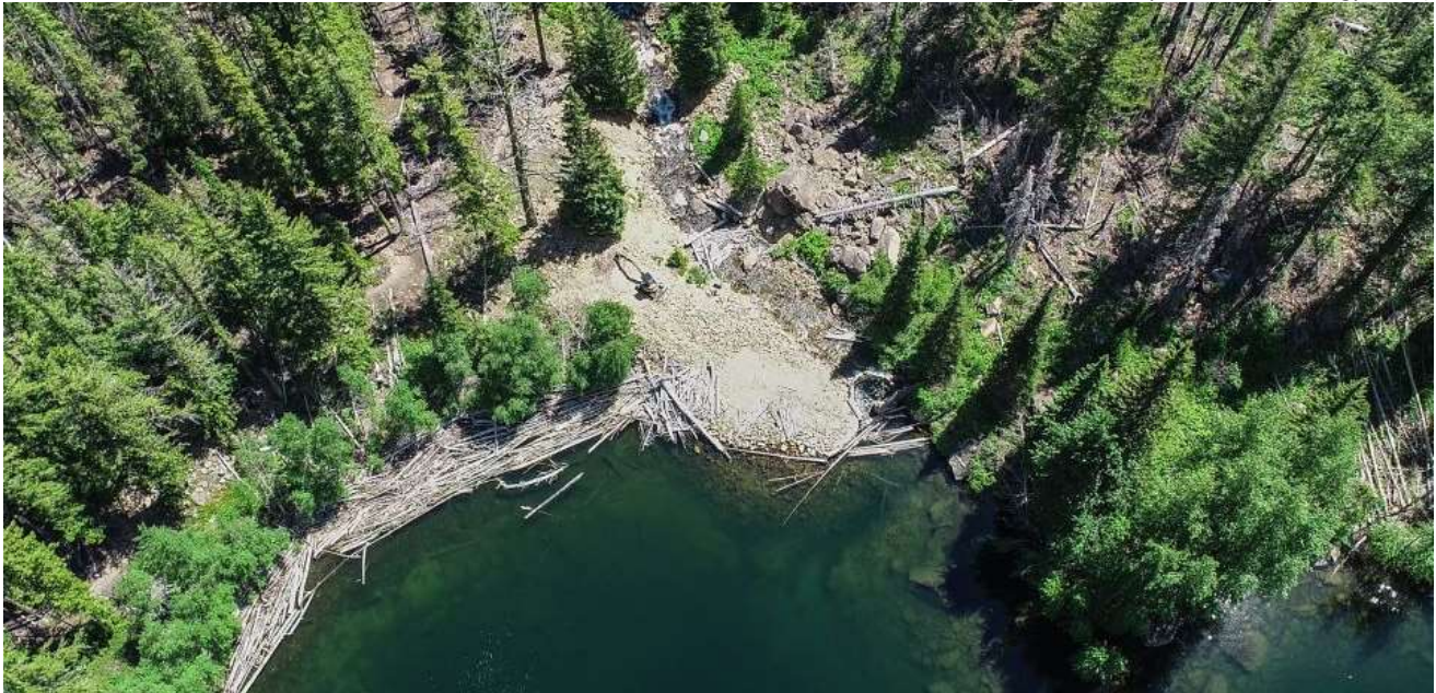
Figure 9-2. Eightmile Lake Dam after 2018 emergency repairs
